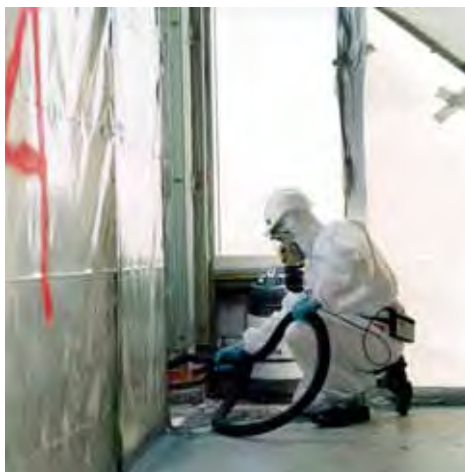
Figure 11: Asbestos removal 1
